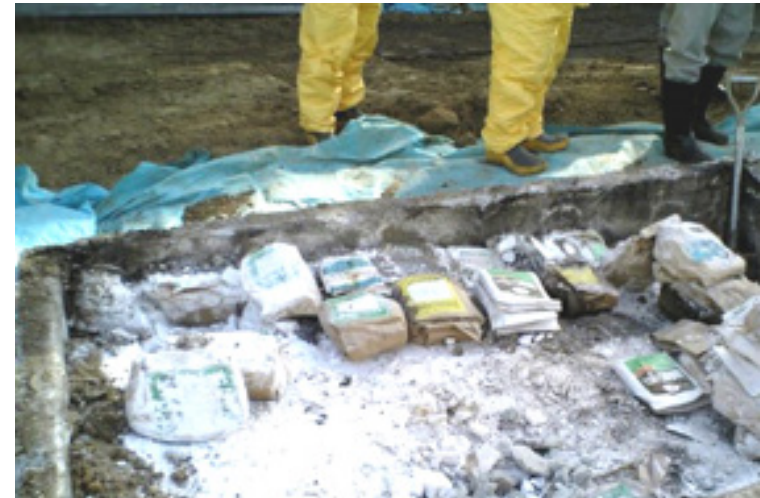
Figure 5: Lindane, DDT, Contaminated Concrete, and Soil Treated at Iga City, Japan
