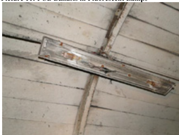
Picture 11: PCB Ballasts in Fluorescent Lamps
