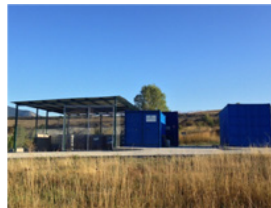
Figure 4: DNAPL Pumping station 1
