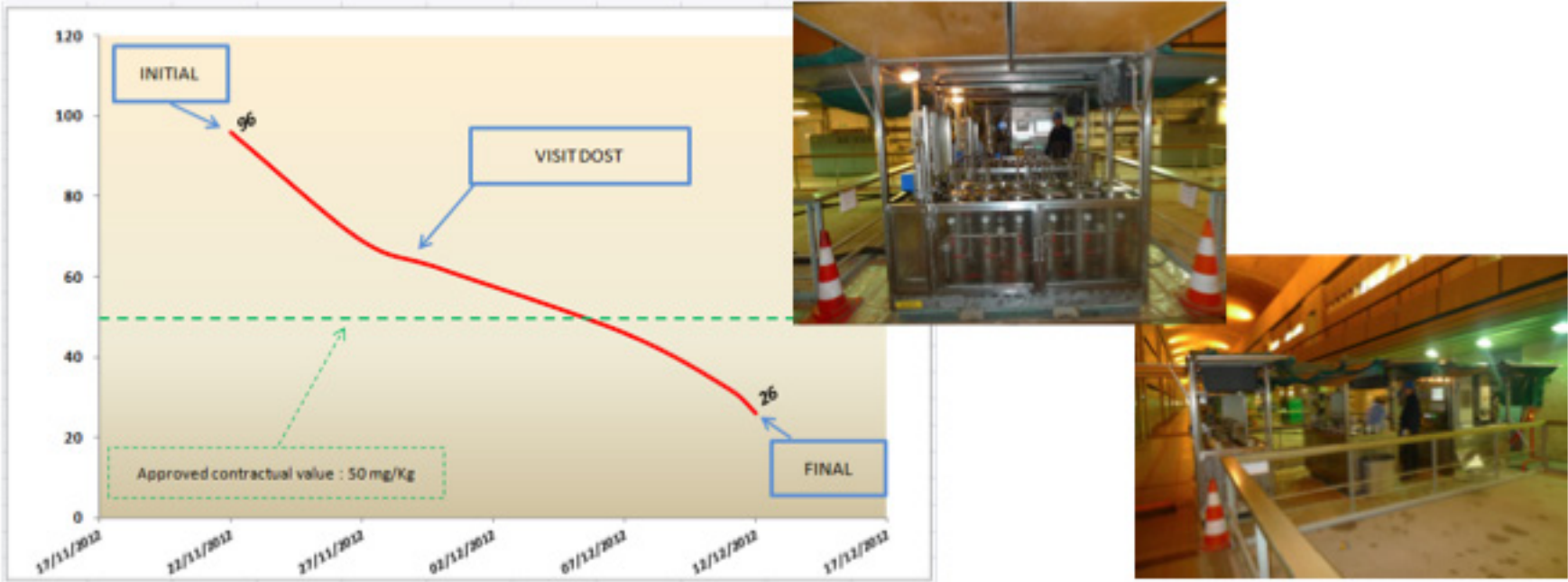
CDP and DMU- Typical applications for power transformers on-site and on-load (Case History France - 2012)
