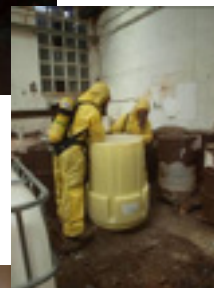
Figure 9 and 10: Repackaging of the drums and liquid waste.
