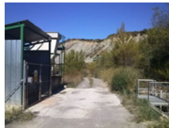
Figure 3: Settling tank (left) and pumping trench
