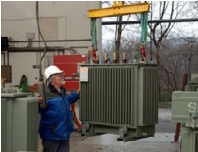
Picture 39: Transformer Maintenance
