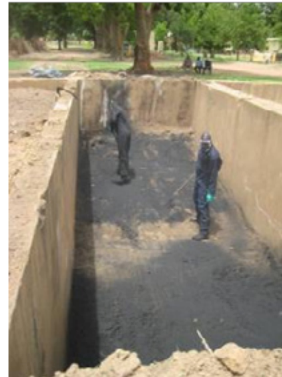
Figure 2: Application of charcoal to prevent leaching
