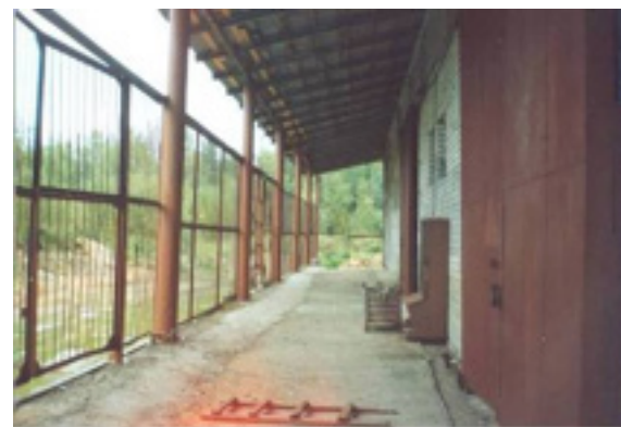
Figure 8: Ruined central warehouse for the storage of pesticides in Syktyvkar
