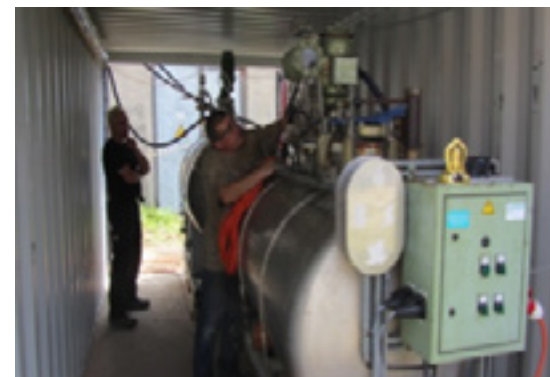
Photo 2: The apparatus for the elimination of the methyl bromide
