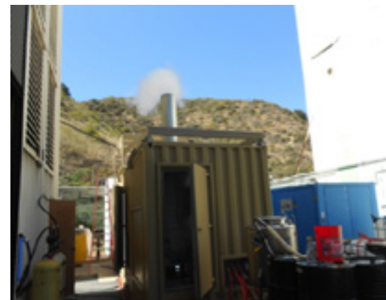
Figure 6: Final Acceptance Test
