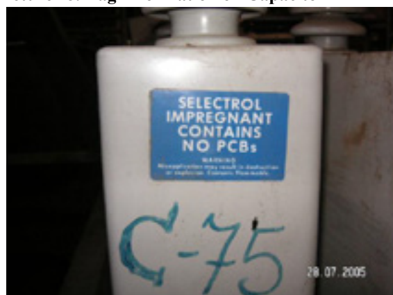
Picture 28: Tag Information on Capacitor
