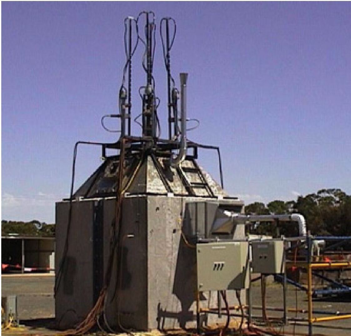
Figure 3: Concrete ICV Treatment Container Used for HCB Treatability Demonstrations
