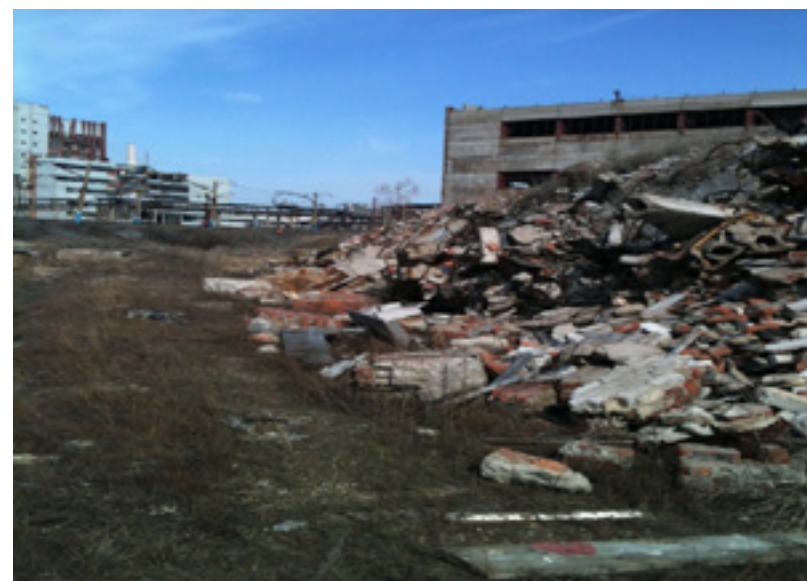
Figure 2: Storing of building breakage of destroyed buildings, 2013
