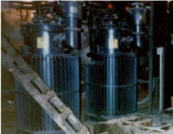
Picture 2: Closed Systems, Transformer
