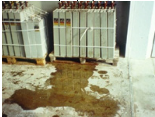
Picture 42: Bad Example II (no tip trays)
