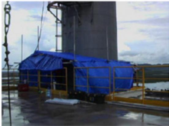
Emission testing facility on kiln stack
