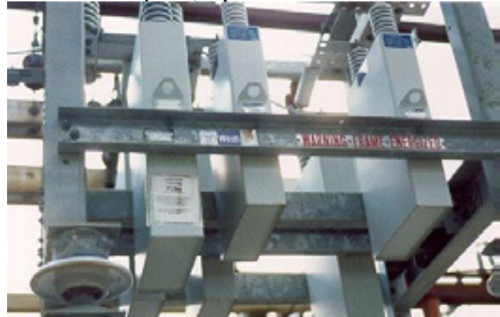
Picture 3: Closed Systems, Capacitors
