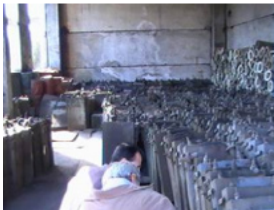
PCB – containing condenser storage in Tajikistan
