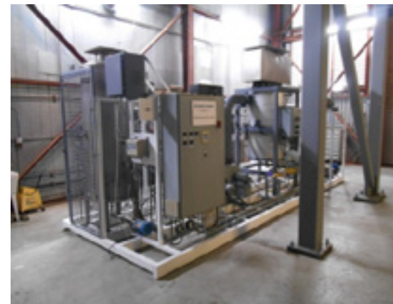
Figure 5: iSCWO Waste Test System
