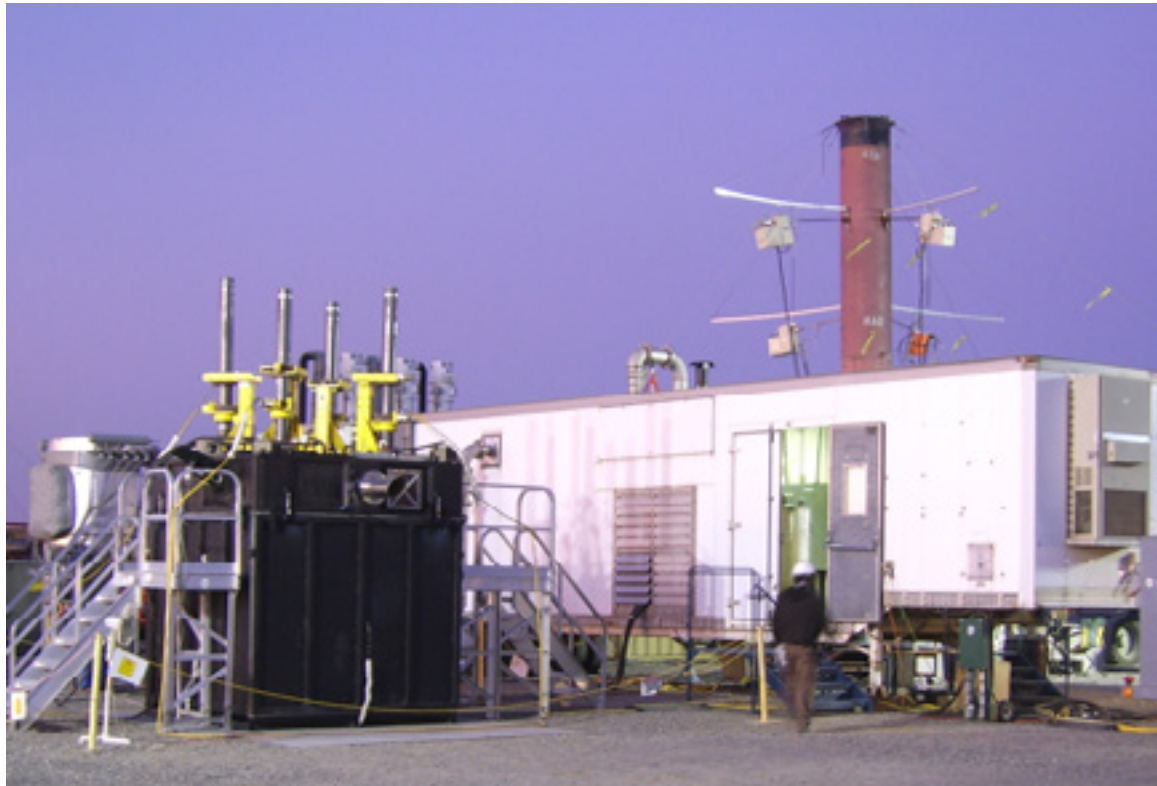
Figure 7: TSCA Permit Renewal PCB Demonstration ICV Container and Process Trailer
