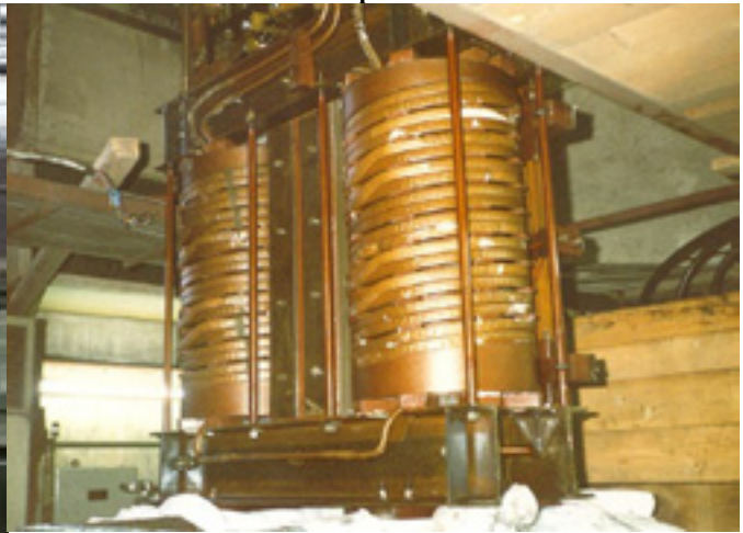
Picture 40: Active transformer part in service station
