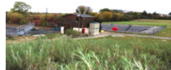
Figure 4: Air filtration system and wastewater treatment plant on site of APROCHIM
