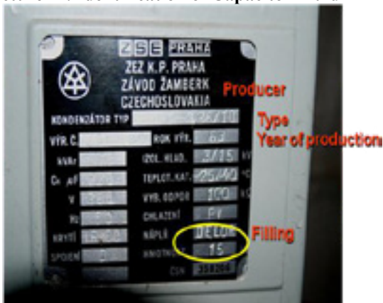
Picture 27: Identification of Capacitor Fluid
