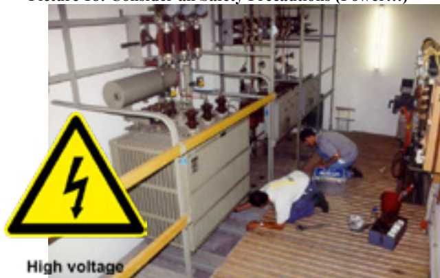
Picture 18: Consider all Safety Precautions (Power!!!)
