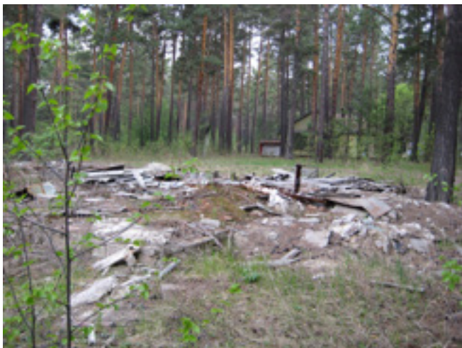
Figure 1: Ruined warehouse on the territory of MUP DSOK “Taiga”
