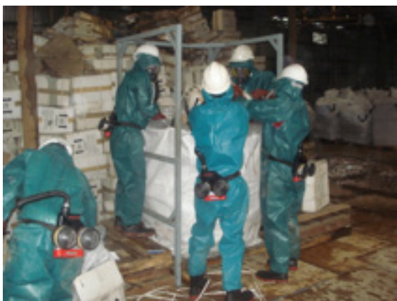
Pictures 1-2: Zoning of the Site area and repackaging works commencement
