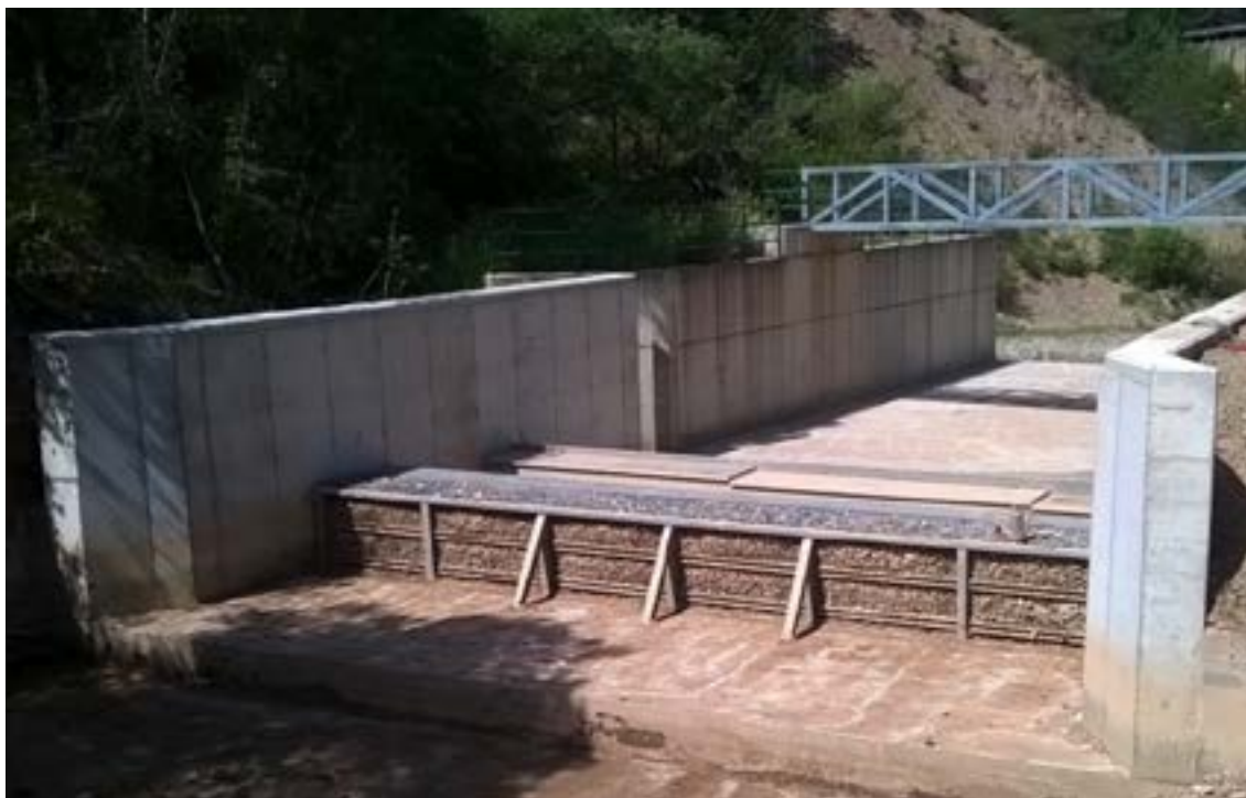
Figure 6. Treatment plant. Decanter and washing deposit and static active charcoal barrier.
