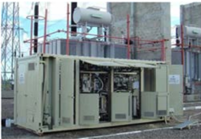
CDP Process ® and DMU- Containerized unit connected with shunt reactor (500 kV) on-load treatment (Brasil 2010)
