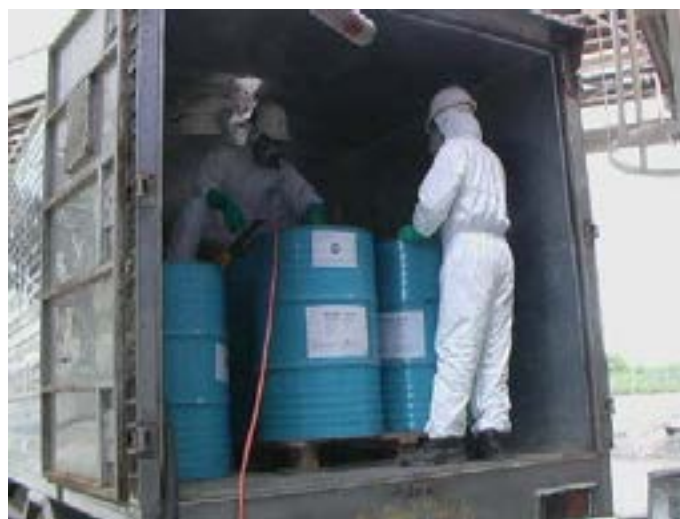
Emptying PCB drums for trial burn
