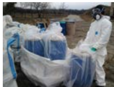
(b) Repacking of the PDC in approved packaging
