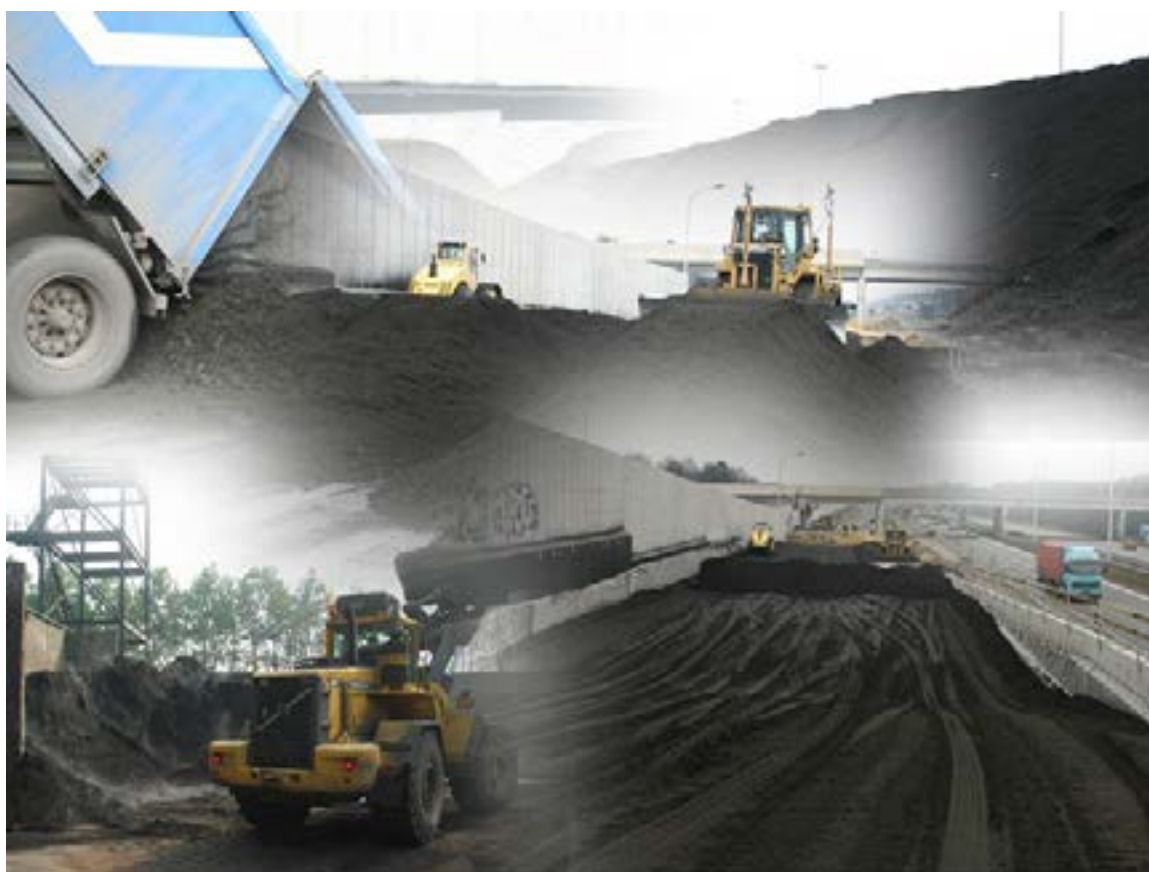
Picture 1. Use of decontaminated soil in civil engineering works
