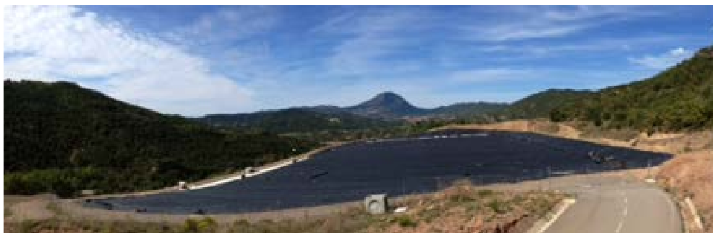
Figure 9. New safety cell sealed temporarily.
