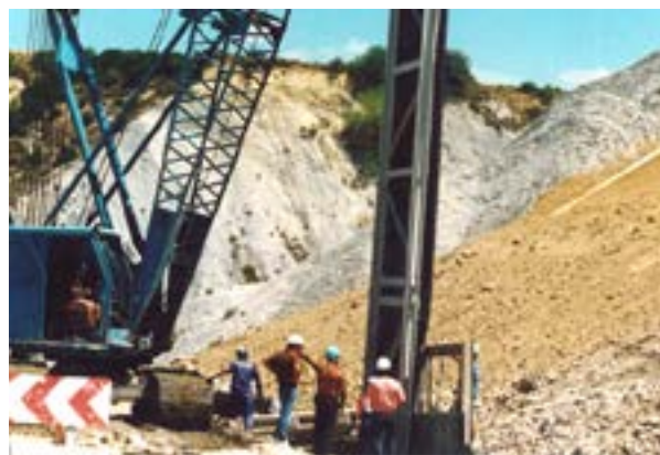
Figure 3. Dumping of excavated waste from the road construction in the lower part of the Sardas landfill site. Sealing and stabilisation of the foot of the landfill.
