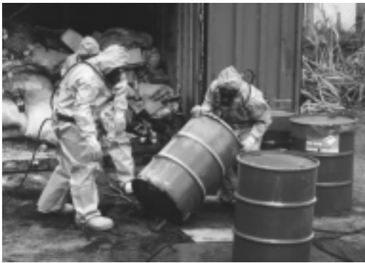
A collection crew overpacking a mixture of products stored in a 20' shipping container at Empresa Nobre in Chimoio, Manica Province.
