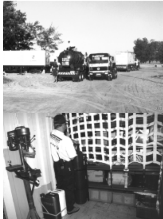
Top Photo: Field re-fuelling of a truck tractor in progress at the campsite in Beira (Sofala Province). Bottom Photo: The mobile workshop and parts
