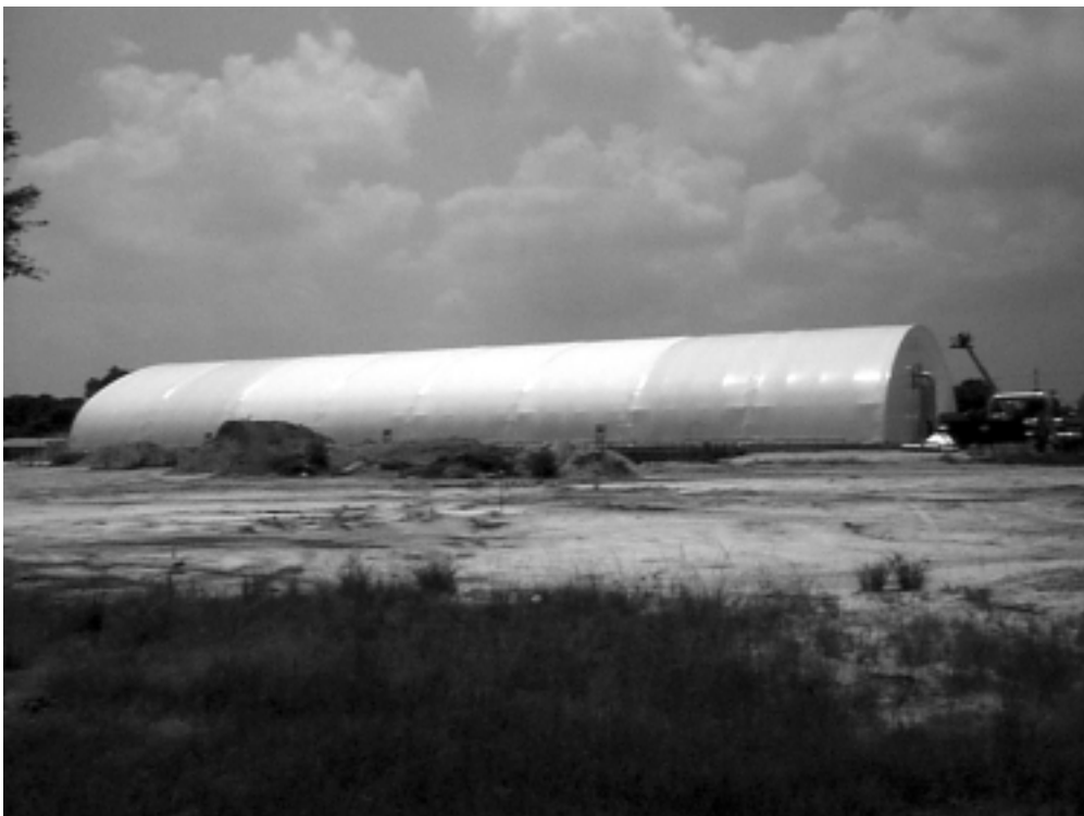
Figure 2. Big top enclosure with odour abatement system
