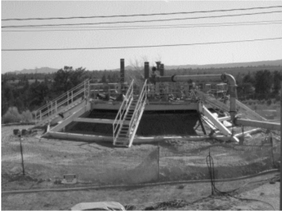
Figure 2. Hood, which is to be placed over the buried waste for in situ vitrification
