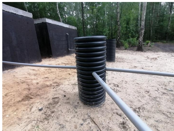
FIGURE 5. THE UNACCEPTABLE CONNECTION BETWEEN TANKS PERFORMED BY PREVIOUS CONTRACTOR
