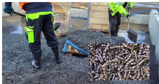
FIGURE 2 FILLING CAST IRON SPONGES INTO MODULE B (+ DETAIL)
